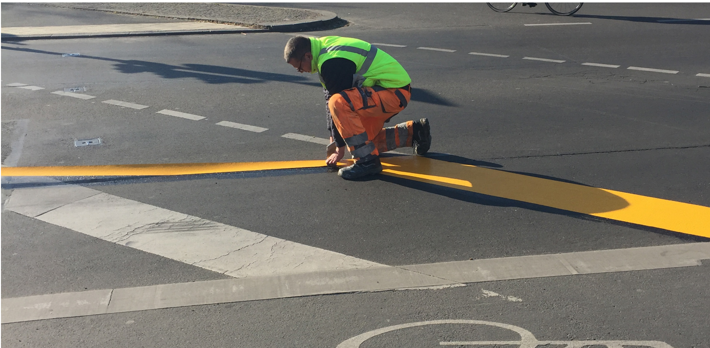
Temporary Measures on Zossener Brücke (Source: Bezirksamt Friedrichshain-Kreuzberg)
