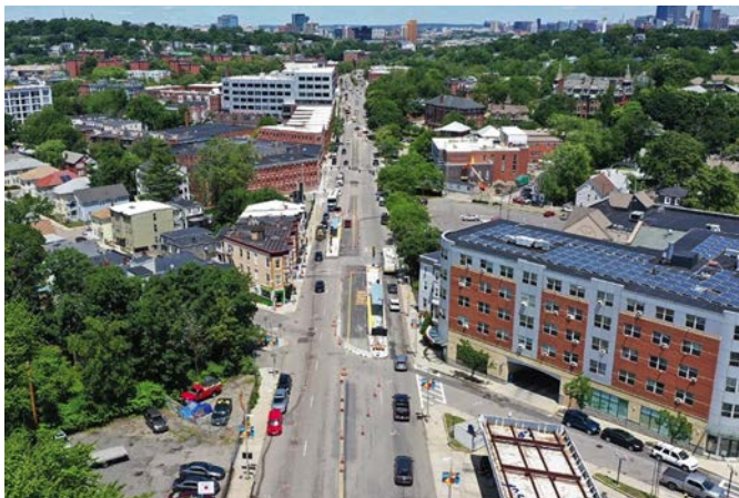
Figure 8-2. Maintenance of traffic plan implementation for Columbus Avenue Bus-Only Lanes Project, Boston, MA.
