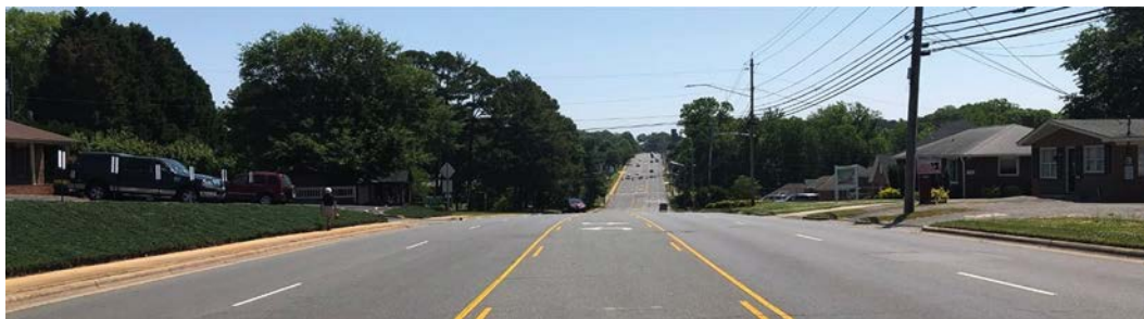
Figure 3-2. Suburban street with missing cross-section components.
