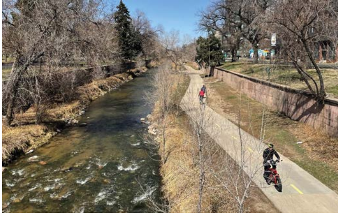
Figure 6-5. Parallel bicycle facilities that facilitate safe travel with minimal route deviation can reduce the cross-sectional width needed to provide safe travel for all roadway users.
