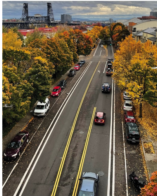
Figure 7-2. Two-lane street with turn lanes in Portland, OR.
