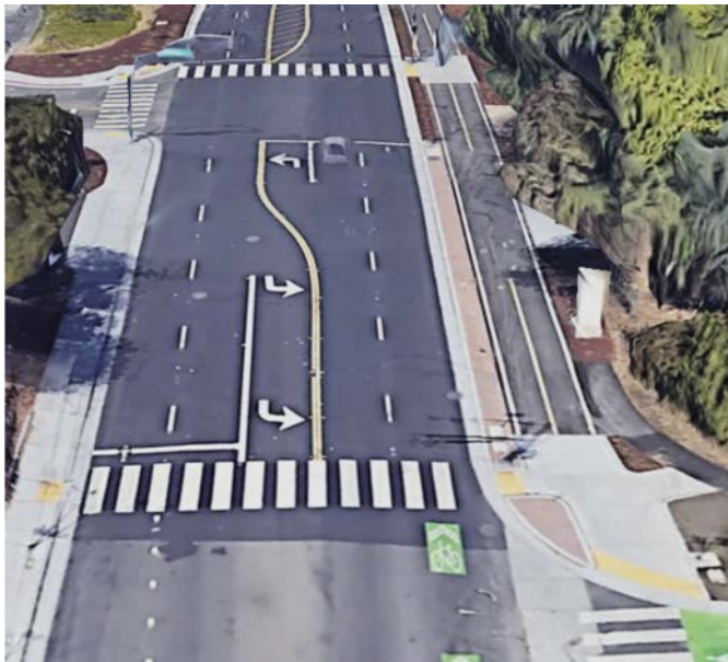
Figure C-1. Aerial imagery showing completed Phase 1 cross section.
