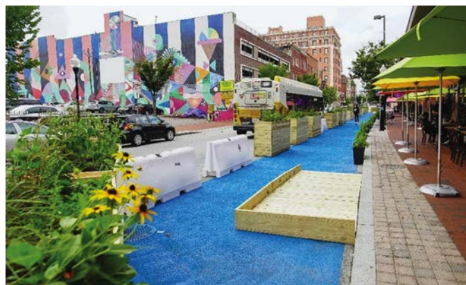
Figure 7-22. A parklet along the curb in Baltimore, MD.
