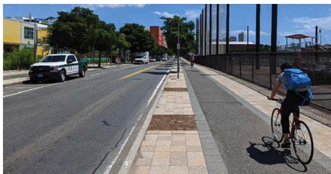
Figure 5-8. A separated bike lane along a distributor street in Cambridge, MA.
