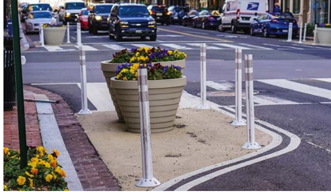
Figure 7-16. A flex post curb extension in Washington, DC.
